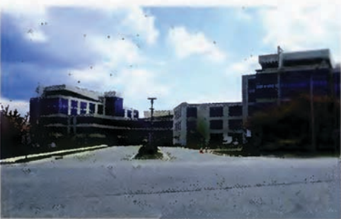
Business park, near Heathrow airport, London
